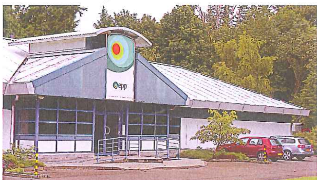
The EPP Environmental Centre, a 1000 m2 laboratory and office facility located in the Bush Estate/Technopole
